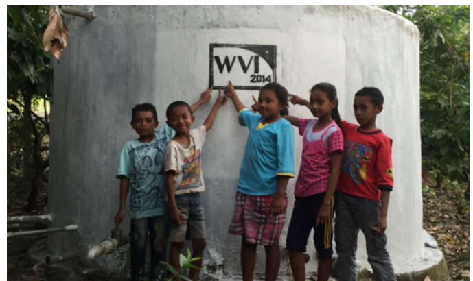
With the construction of a water tank, pipes and taps, these children no longer need to travel great distances through dangerous trails to fetch water.
