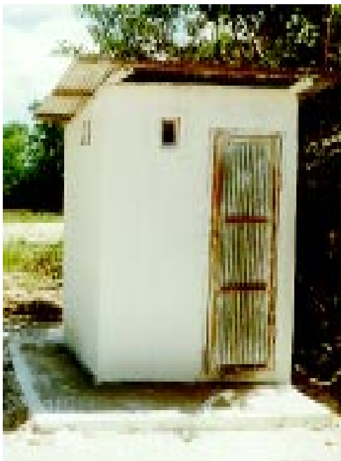
The 1st newly-constructed latrine in the village
